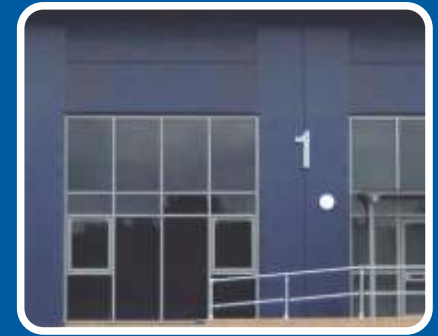
Low Rise Curtain Walling
