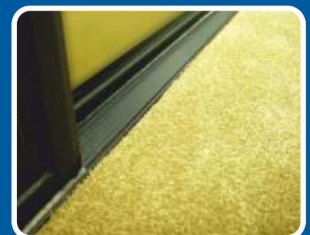
Flush Internal Floor Level
