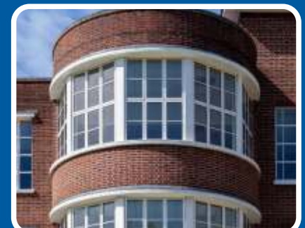
Meets Building Regs
